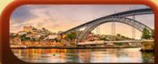
DOM LUIS I BRIDGE
